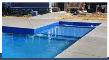
**Note:** the sun ledge area only needs to be excavated 22" deep. ALPSMfg will supply 22" steel walls and bracing for the side walls and ship a complete sun ledge kit including all bracing.
