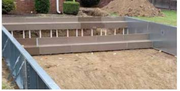
This sun ledge installation has the entire sun ledge excavated revealing the PVC pipe used to level the steps at the end of the pool.
